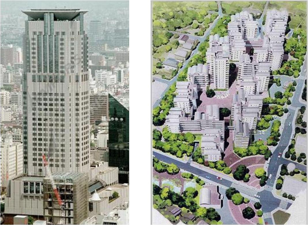
Figure 3. Left: Applause Building in Osaka, with a hybrid control system moving an heliport structure at the top. Right: sketch of the complex of 21 six- to fourteen-storey buildings erected on a unique “artificial ground” isolated at Sagami-hara (Tokyo area) with 48 lead rubber bearings (LRBs), 103 sliding devices (SDs) and 83 ball bearings.
