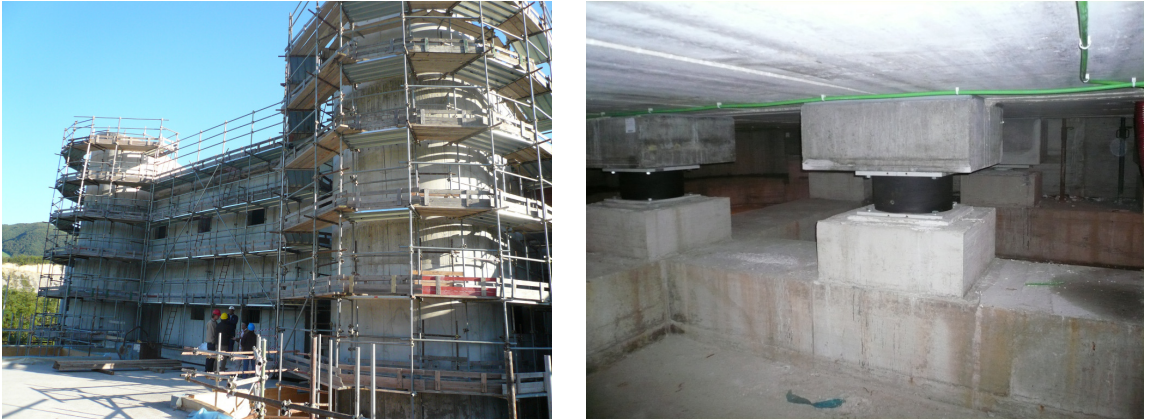
Figure 38. The new school in Marzabotto (Bologna), in seismic zone 3, erected on HDRBs and SDs. Its safety was certified by A. Martelli in September 2010.
