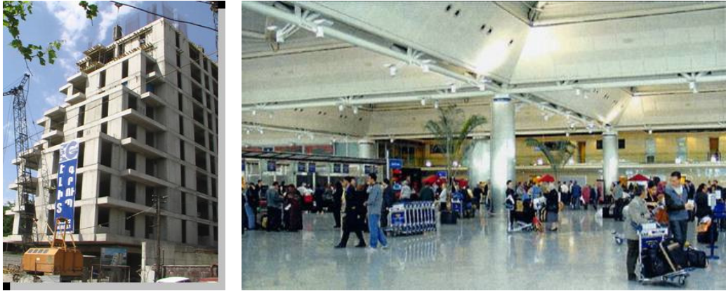
Figure 54. Left: the 15-storey Cascade multifunctional complex, isolated in Yerevan by MDRBs in 2006. Construction of even taller buildings is in progress. Right: the roof of the new Ataturk Airport in Istanbul, isolated by means of 100 FPS devices in 1999.
