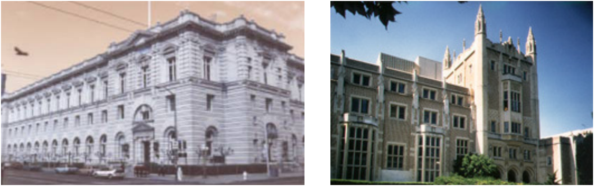
Figure 23. Further US building retrofits with SI. Left: San Francisco Court of Appeal, retrofitted with FPS. Right: Kerckhoff Hall at the University of California, Los Angeles (total living area = 8,300 m 2 , 6 storeys).
