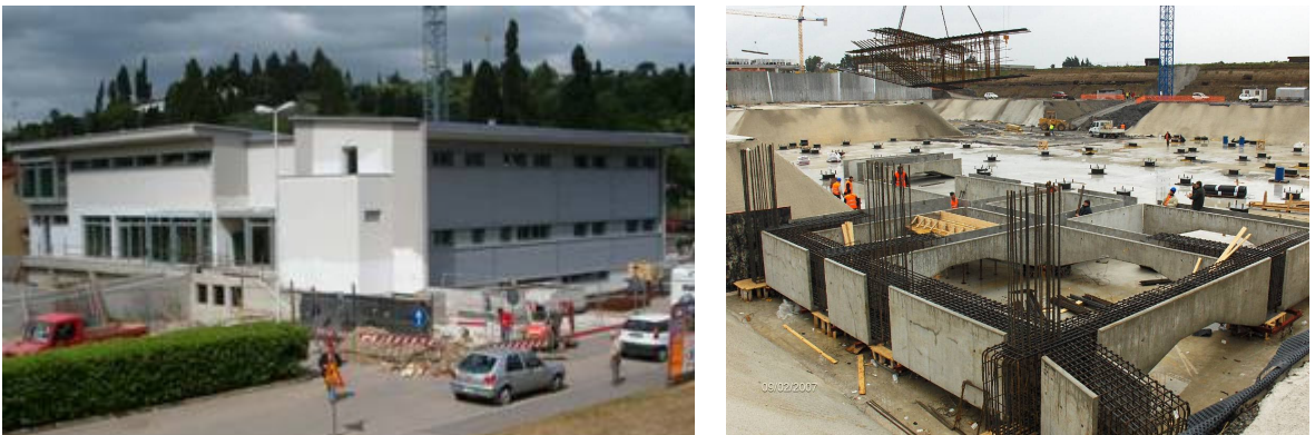
Figure 41. Left: Headquarters of the association Fratellanza Popolare – Croce d’Oro in Grassina (Florence), in seismic zone 2, isolated by means of SDs and VDs; it is a L-shaped building to be used for civil defense, designed by the GLIS board and ASSISi member S. Sorace of the University of Udine and certified as safe by A. Martelli in 2007. Right: NATO Centre in South Naples, in seismic zone 2 (399 HDRBs and 20 dissipative SDs), during construction in 2007.
