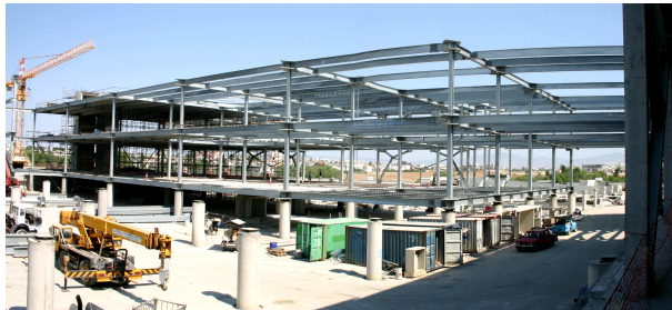
Figure 60. The Shakolas Park Commercial Centre at Nicosia (Cyprus), designed by the Italian GLIS board and ASSISi member G. C. Giuliani and his son of Redesco (Milan), formed by two buildings with mixed r.c. and steel structure, with 164 Italian HDRBs installed at top of the basement columns, during construction in 2007.
