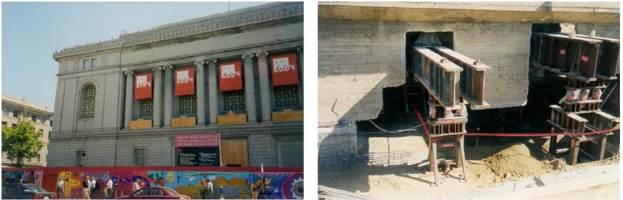
Figure 21. Asian Art Museum in San Francisco, during its seismic retrofit (with cut of the foundations and insertion of HDRBs) performed according to the design of the Italian architect Gae Aulenti (late 1990s).
