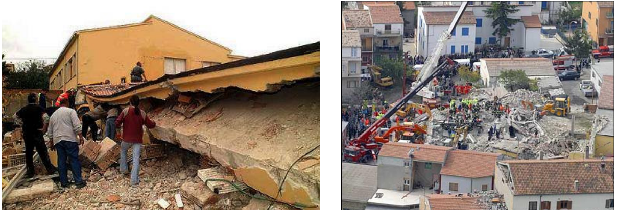
Figure 24. Collapse of the Francesco Jovine primary school in San Giuliano di Puglia (Campobasso) during the 2002 Molise and Puglia earthquake, and search for survivors amid the debris.
