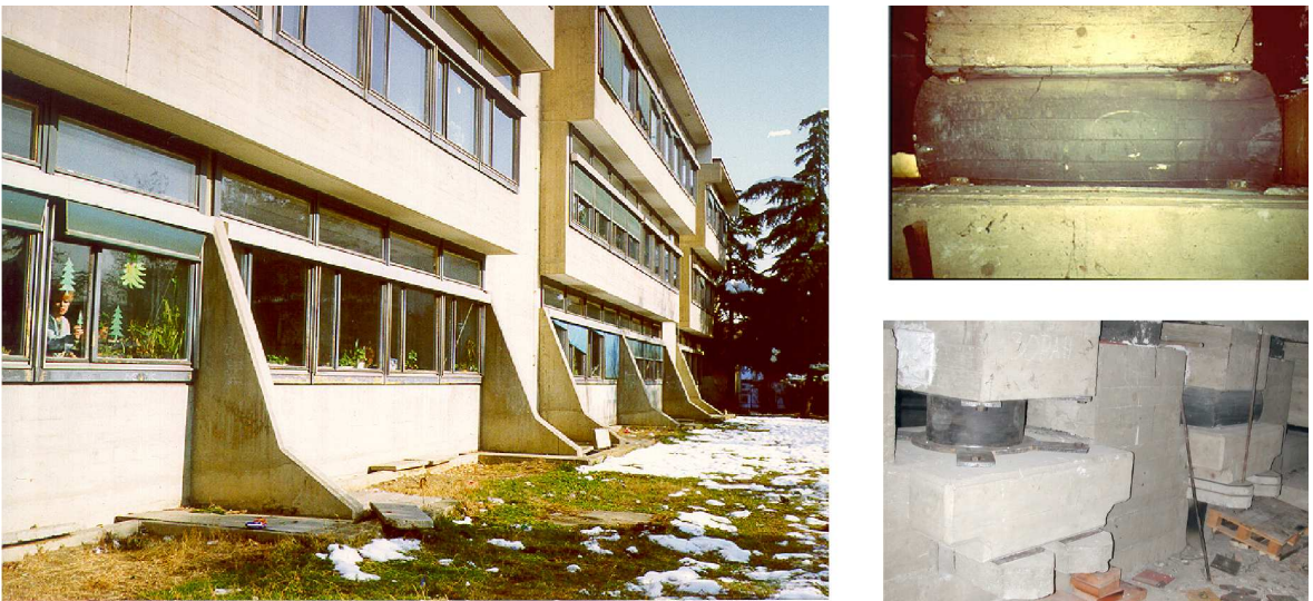
Figure 65. Left: the isolated Pestalozzi school at Skopje (Macedonia), built in the 1960s. Top right: a very degraded original low damping rubber bearing (LDRB). Bottom right: a new HDRB, next to original LDRBs yet to be replaced.
