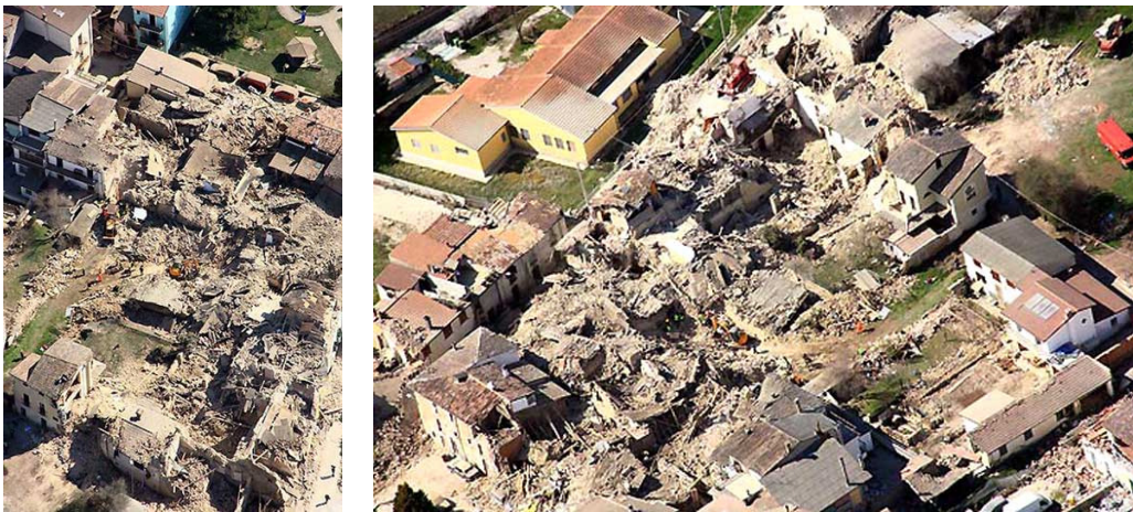
Figure 26. L'Aquila (April 2009): aerial views of some parts of the town where buildings collapsed or were heavily damaged.
