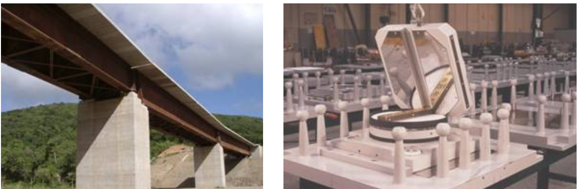
Figure 64. The The Caracas – Tuy Medio railway in Venezuela (26 isostatic span viaducts, overall length = 7,775 m, 217 spans), protected by over 1,500 isolators manufactured in Italy in 1999–2003.
