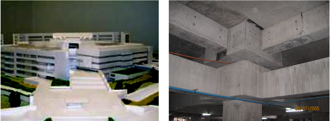
Figure 63. The new building of the Hospital Militar de Santiago (80,000 m 2 ), in the community of La Reina, under construction in 2006. It is equipped with 114 HDRBs and 50 LRBs.
