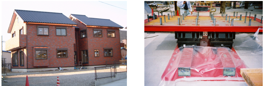
Figure 6. A Japanese private house protected by an SI system formed by steel sphere recirculation isolators, viscous dampers (VDs) and recentering devices.
