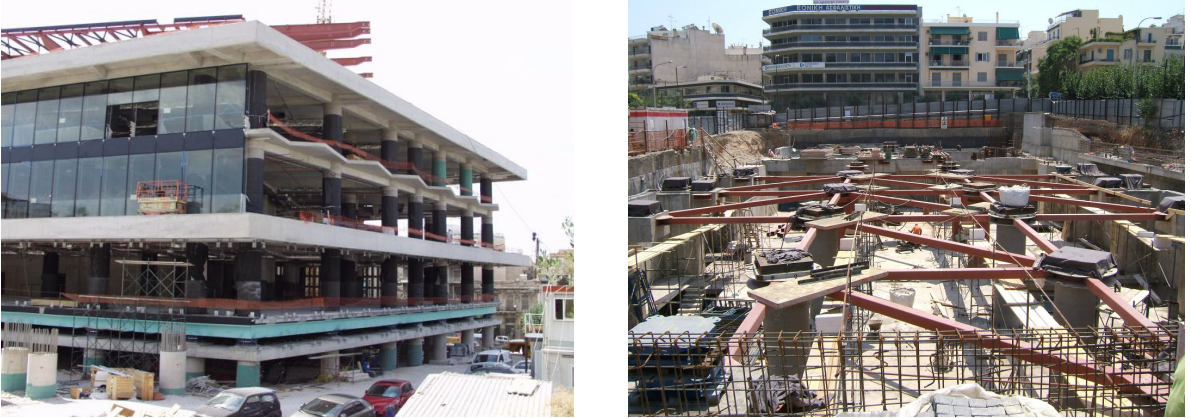
Figure 59. Left: the Onassis Centre in Athens, with the Acropolis Museum, isolated in 2007 by 94 German SIP devices in 2006 (left). Right: the Onassis House of Letters and Fine Arts, during its construction, again with German SIP devices.
