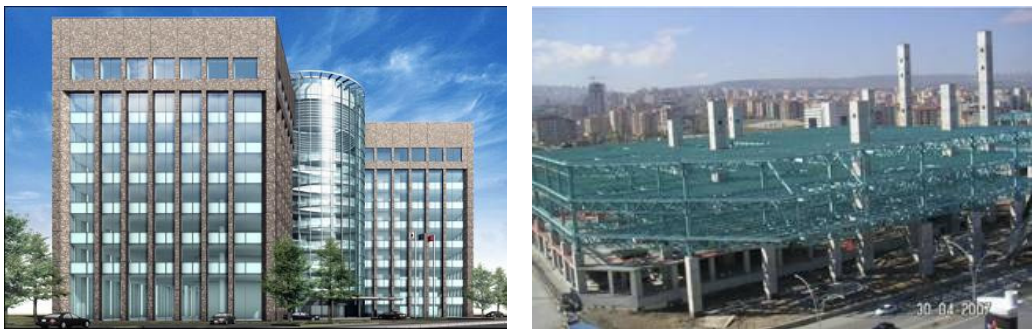
Figure 55. Isolated buildings in Turkey. Left: the T.E.B. Headquarters, a building which was under construction on 87 LRBs and LDRBs in Istanbul in 2006. Right: Söğütözü Congress and Commercial Centre in Ankara, isolated using 105 SIP devices manufactured in Germany in 2007.
