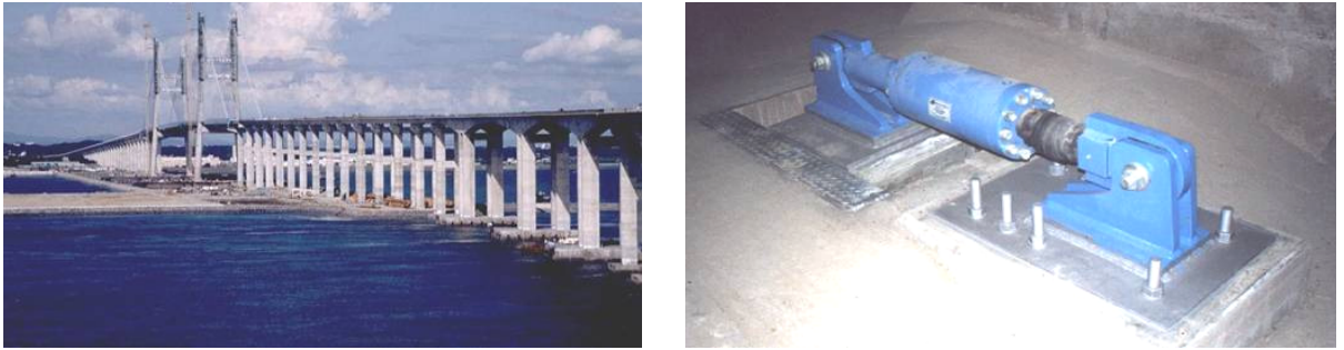
Figure 49. Approaches of the Seo-Hae Granel Bridge in South Korea (overall length 5820 m, height of piles 12–60 m), which were retrofitted by means of 54 Italian VDs ( K = 100 \text{ kN/mm} ) in 2000–2001.
