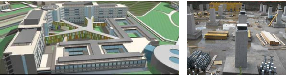
Figure 34. Sketch of the new isolated Del Mare Hospital, during its construction in Naples, nowadays in seismic zone 2, and view of some of its 327 HDRBs. Several new Italian hospitals being or to be erected in seismic areas now include the use of SI.
