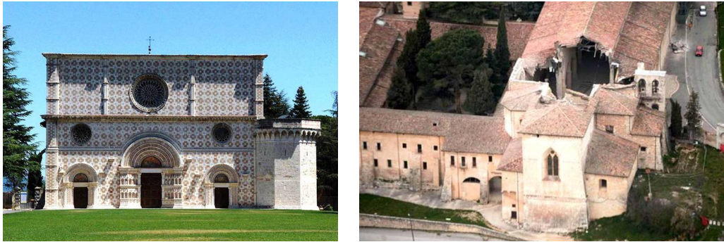
Figure 28. The Cathedral of Santa Maria di Collemaggio, a rare example of Abruzzo Romanesque style, prior to the earthquake, and the collapse of the roof of its baroque (not yet retrofitted) part. The façade, which had been protected by some EPDs installed on the roof some years earlier (see Figure 45 ), survived the earthquake; however, a steel scaffold, previously erected for an already planned retrofit, certainly helped.
