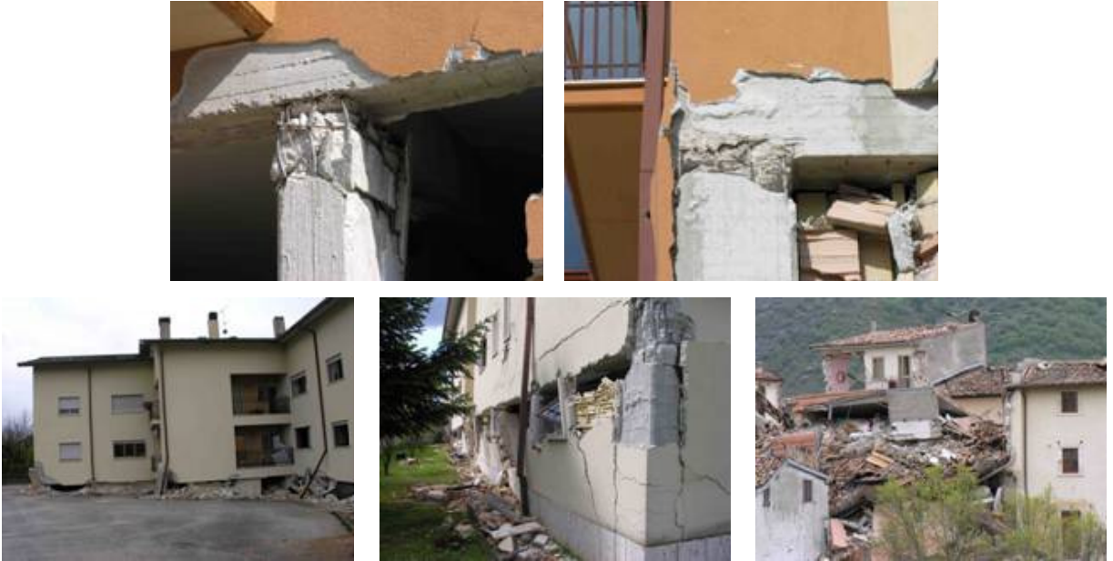
Figure 30. L'Aquila (April 2009): partly collapsed and heavily damaged private buildings. Note in particular the heavily damaged beam-column joints (top row).
