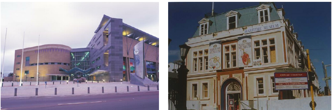
Figure 52. Wellington, New Zealand: the isolated Te Papa Museum (left) and the Maritime Museum (right), retrofitted with SI in 1993.
