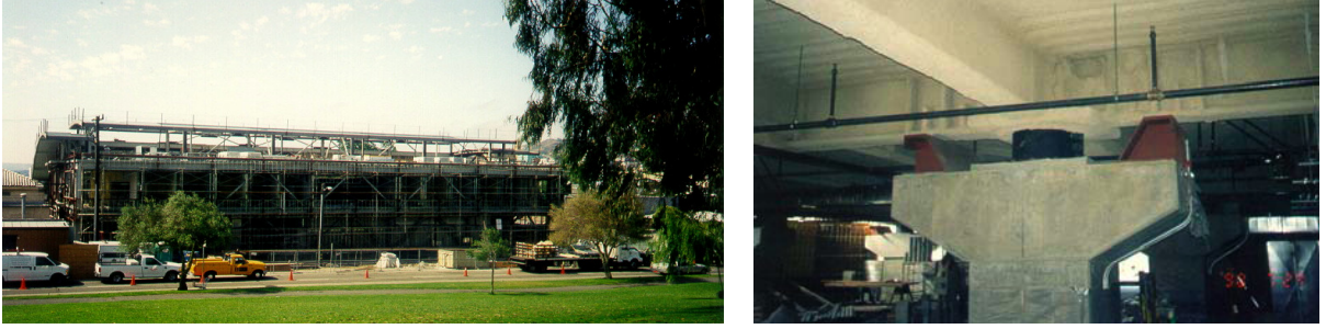
Figure 20. Left: construction of the 911 Emergency Communications Center in San Francisco, designed to withstand earthquakes to magnitude M = 8.3 . Right: view of one of its RBs and the fail-safe system (late 1990s).
