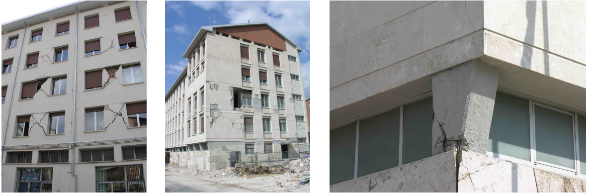
Figure 32. L'Aquila (April 2009): headquarters of ANAS (the Italian agency for road construction and maintenance), which suffered mainly nonstructural damage (with the exception of two pillars, which, however, are reparable — see right. Retrofit by means of SI was possible and was suggested for this building.
