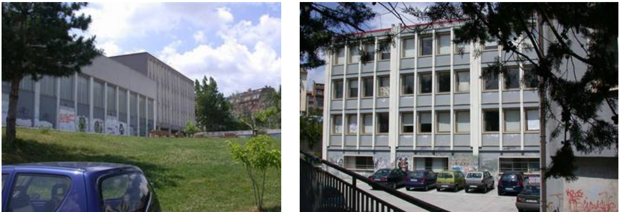
Figure 39. Romita High School for scientific studies of Campobasso (hosting about 1,300 students), in seismic zone 2, which was at last partly demolished and is now being rebuilt with SI, due to its very poor concrete quality (as demonstrated by an ENEA study performed after the 2002 Molise and Puglia earthquake). Safety of the new seismically isolated buildings will be certified by A. Martelli.
