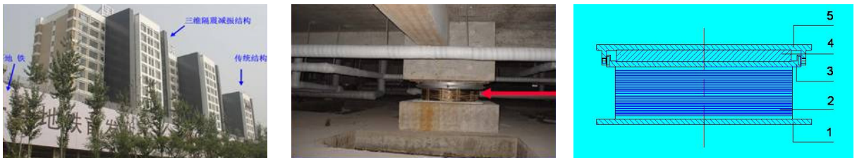
Figure 12. Left: new Chinese buildings protected at Guangzhou by 3D RBs from both horizontal seismic vibrations and vertical traffic vibrations. Center: one of the 3D RBs. Right: its sketch (4 = vertical element). Similar applications exist in Beijing.
