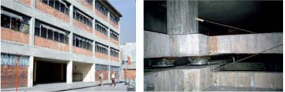
Figure 56. The Legaria Secondary school at Mexico City (first Mexican application of SI, performed in 1974) and one of its rolling SI devices, developed in Mexico.
