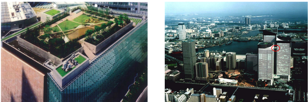
Figure 7. Left: “green mass damper”, used as the TMD of a 45 m tall building of the Keyaki-zaka residential complex, in Tokyo. The garden base is 1 m thick, weights 3,650 t, or 8% of the building mass, and is supported by 46 rubber bearings (RBs) and 22 visco-elastic dampers (VEDs). Right: ADB between Japanese high-rise buildings.
