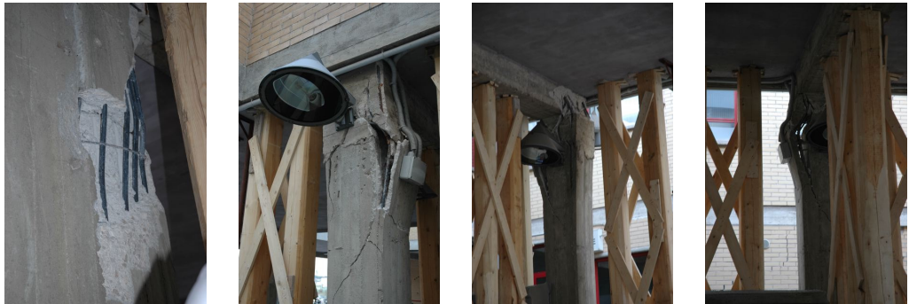
Figure 29. L'Aquila (April 2009): pillars in the San Salvatore Hospital, heavily damaged due to very inadequate steel reinforcement and poor concrete quality (no inert materials are visible in the upper part of the pillar).
