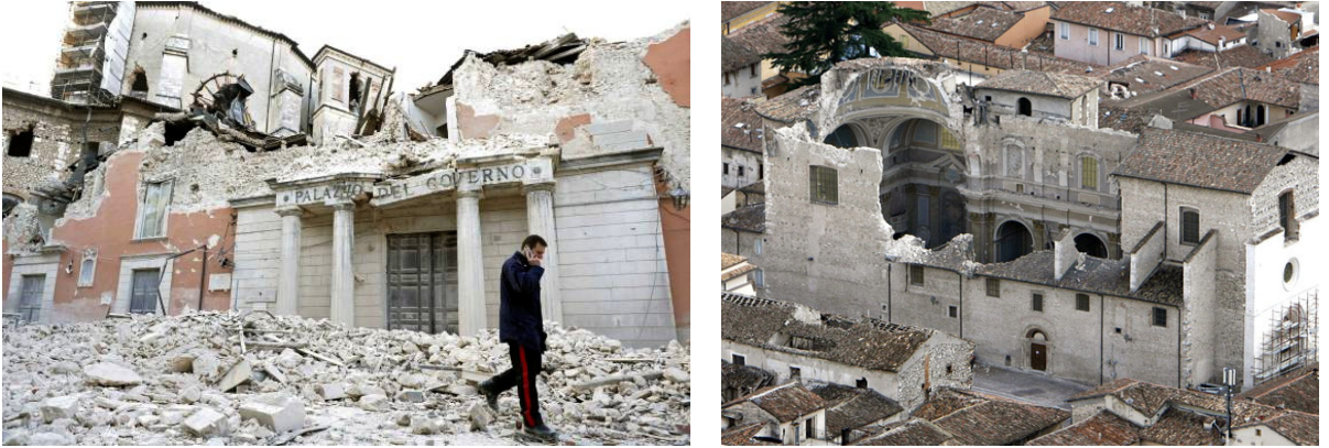
Figure 27. L'Aquila (April 2009): collapse of the Prefettura building (provincial headquarters of the national government) and the Santa Maria Paganica Church (right).
