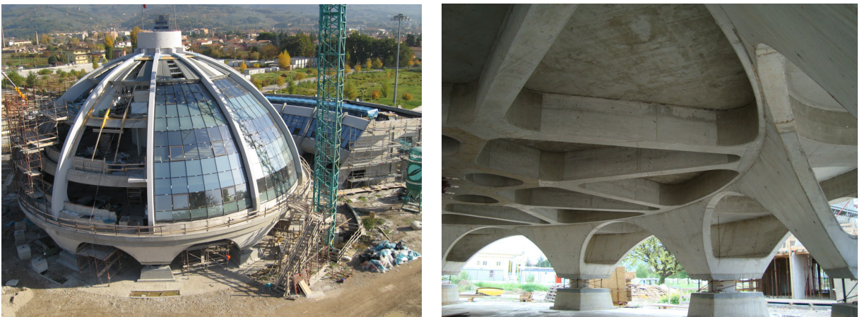
Figure 35. The Emergency and Management Operative Center of the new Civil Defense Center of Central Italy in Foligno (Perugia) was designed by the GLIS board and ASSISi member A. Parducci of e-Campus University. Their safety will soon be certified by A. Martelli. The photo on the left shows in the foreground the main building, which is being erected on ten HDRBs of 1 m diameter, two of which are seen on the right, with provisional protective covers. Also seen on the left is the adjacent service building, isolated by HDRBs and SDs. The Foligno Center will include at least seven isolated buildings, three of which have already been completed. Its site was reclassified from seismic category 2 to seismic zone 1 in 2003, but no design changes of the structures and foundations were necessary, thanks to SI. An increase in the diameters of isolators was sufficient, as demonstrated by a study performed by ENEA.
