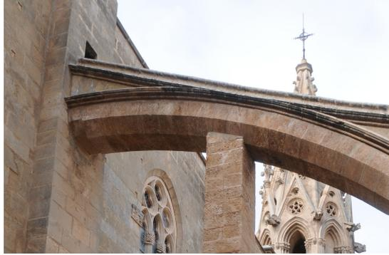
**Figure 14.** Sliding in the upper flying buttress B6N. Note that the sliding is not between the wall and the first voussoir, but between first and second voussoirs [Photo: Roland Wiczorek, BTU Cottbus-Senftenberg].
