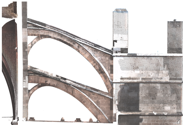
Figure 16. Orthophoto of south flying buttresses B1 (based on the cloud of points by Rex Haberland).
