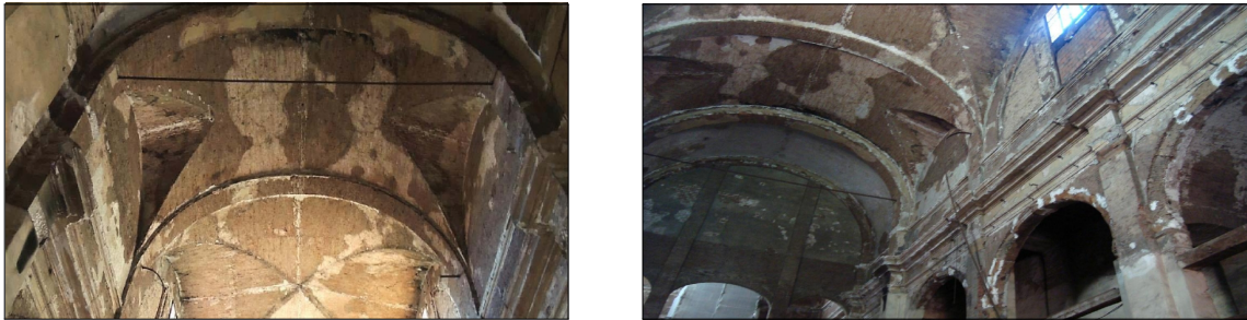
Figure 4. Intrados of the barrel vault with lunette in the San Barbaziano church.
