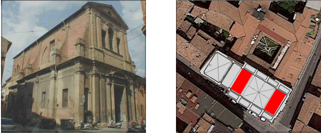
Figure 2. The San Barbaziano church: external view (left) and ground level plan (right).
