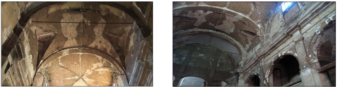
Figure 4. Intrados of the barrel vault with lunette in the San Barbaziano church.
