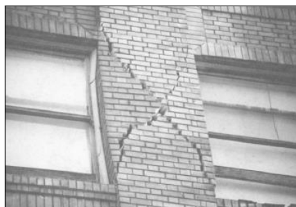
Figure 5. The typical X-shaped cracking pattern occurring in a wall pier.
