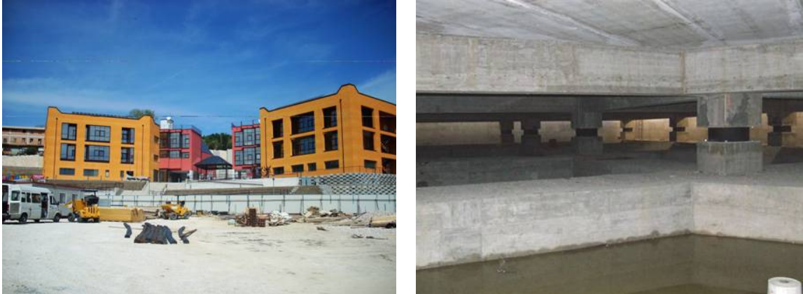
Figure 36. The new Francesco Jovine primary school and Le Tre Torri Professional and University Centre, erected in San Giuliano di Puglia (seismic zone 2 since 2003) on a single seismically isolated slab, and its SI system (61 HDRBs and 12 SDs) during construction. The isolators were donated by the Italian ALGA, FIP Industriale and TIS manufacturing companies. The SI design is by a team of experts coordinated by the GLIS and ASSISi member P. Clemente of ENEA, with tests done by the University of Basilicata. Safety was certified by A. Martelli and GLIS member C. Pasquale in September 2008.
