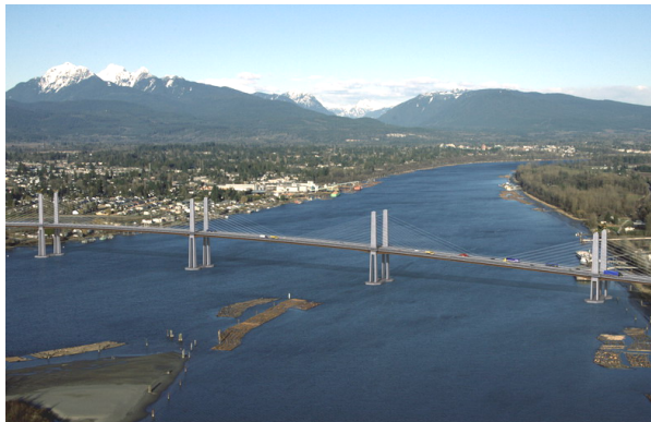
Figure 62. Golden Ear Bridge (Canada), isolated in 2007 by means of Italian CSS devices.
