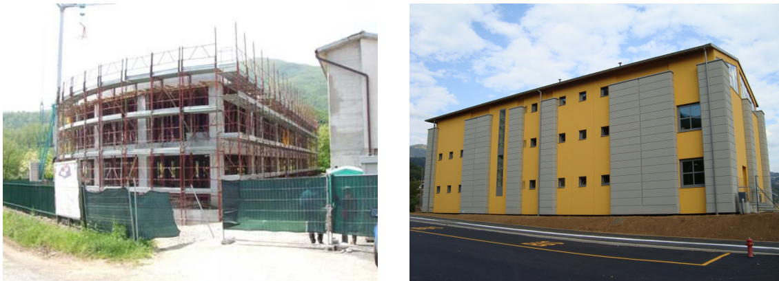
Figure 37. The first new school building of Mulazzo (Massa Carrara), protected by LRBs and SDs (right) and the new primary and secondary school of Galliciano (Lucca), protected by HDRBs and completed in September 2009. They are two of the 5 schools rebuilt or being rebuilt with SI in Tuscany, in seismic zones 2. Safety of the Mulazzo school will be certified by A. Martelli, that of the Galliciano was certified by A. Parducci.
