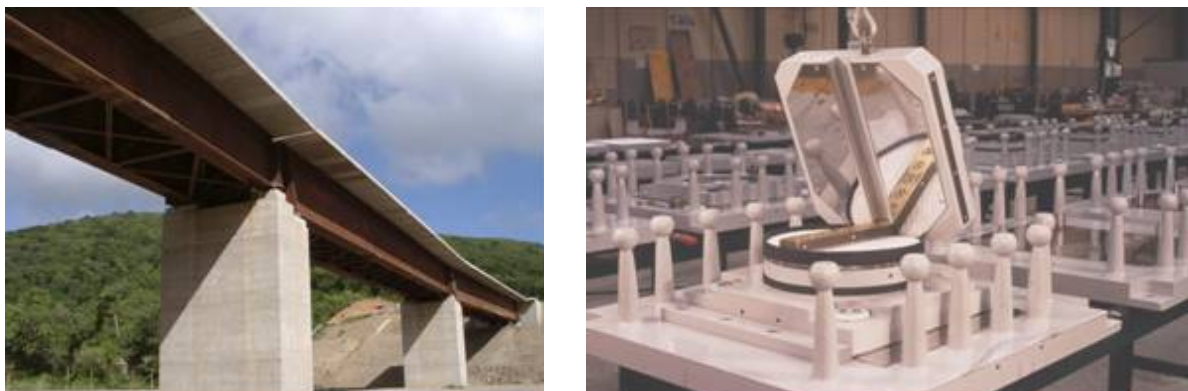
Figure 64. The Caracas – Tuy Medio railway in Venezuela (26 isostatic span viaducts, overall length = 7,775 m, 217 spans), protected by over 1,500 isolators manufactured in Italy in 1999–2003.
