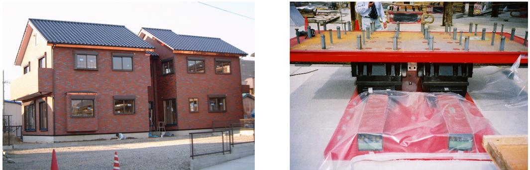
**Figure 6.** A Japanese private house protected by an SI system formed by steel sphere recirculation isolators, viscous dampers (VDs) and recentering devices.
