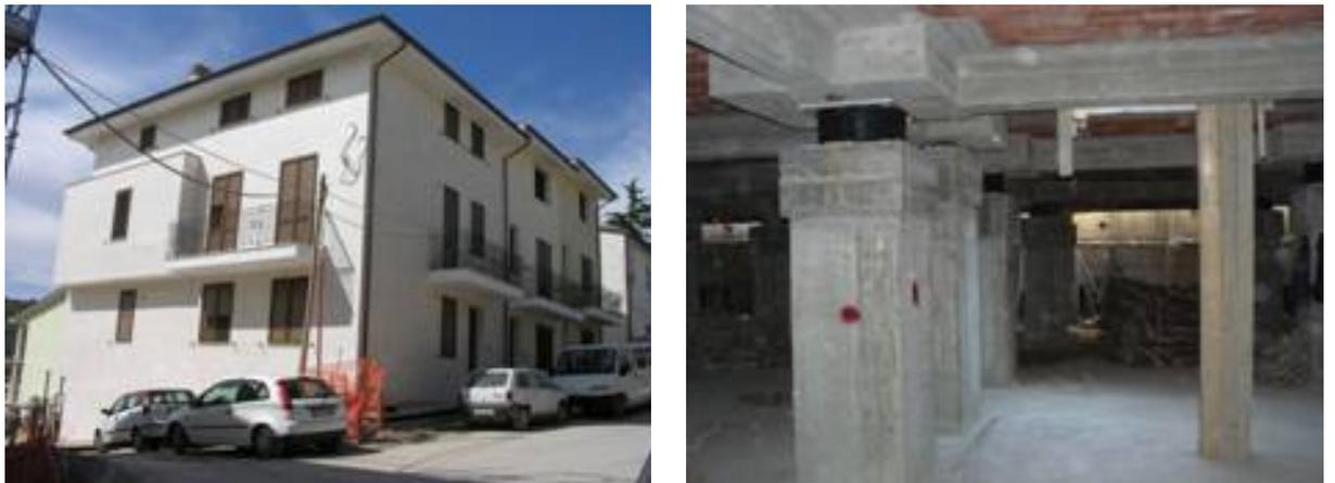
**Figure 43.** Left: residential building in San Giuliano di Puglia, isolated by 13 HDRBs and 2 SDs with the collaboration of ENEA, completed in 2007. Right: SI formed by LRBs and SDs of an 8-storey building under construction at Messina, in seismic zone 1; its safety will be certified by A. Martelli.
