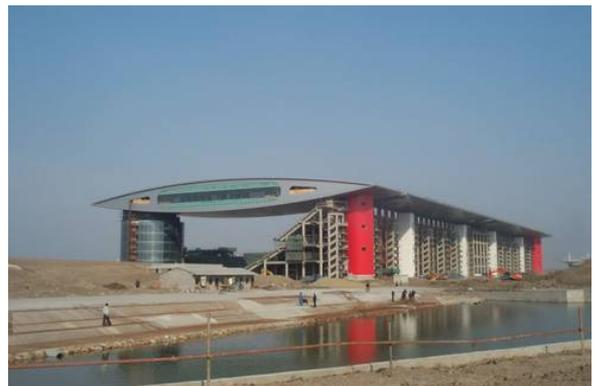
**Figure 16.** Left: Chinese stadium (23,000 m<sup>2</sup>) protected by RBs and VDs, for which SI reduced the seismic response by a factor of 4.2. Right: and roof SI of the News Centre and Restaurant of Shanghai F1 Autodrome.
