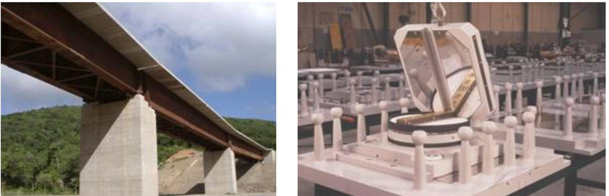
**Figure 64.** The The Caracas – Tuy Medio railway in Venezuela (26 isostatic span viaducts, overall length = 7,775 m, 217 spans), protected by over 1,500 isolators manufactured in Italy in 1999–2003.
