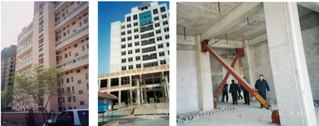
**Figure 11.** The tallest seismically isolated Chinese building (19 storeys), erected at Taiyuan City, in Northern China (left), and a Chinese high-rise building protected by VDs (center and right).
