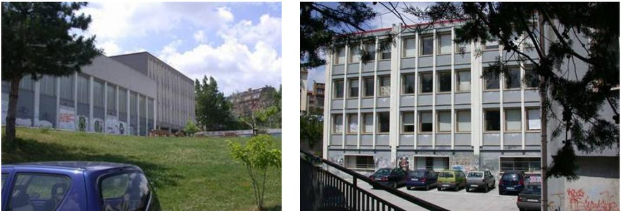
**Figure 39.** Romita High School for scientific studies of Campobasso (hosting about 1,300 students), in seismic zone 2, which was at last partly demolished and is now being rebuilt with SI, due to its very poor concrete quality (as demonstrated by an ENEA study performed after the 2002 Molise and Puglia earthquake). Safety of the new seismically isolated buildings will be certified by A. Martelli.
