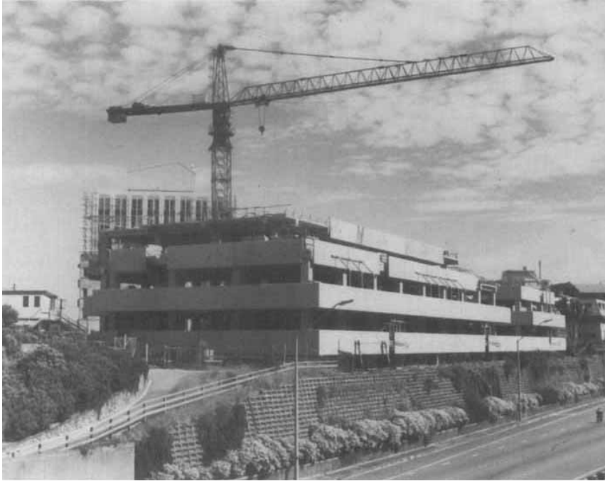
Figure 13. Wm Clayton Building as at March 1981
